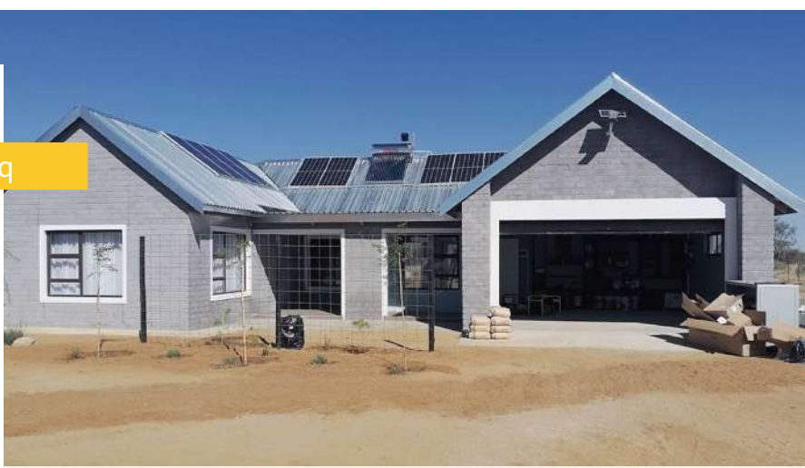
UU 48-350 LiFePO 4 Battery Solar Panel Inverter
